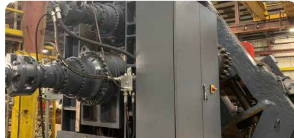
UPGRADE TO NC
