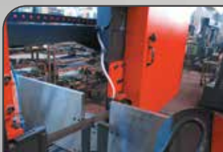
33- PROXIMITY SWITCH FOR SENSING BLADE SLIPPAGE
