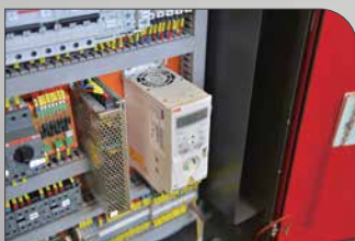
13-INVERTER (VARIABLE SPEED)
