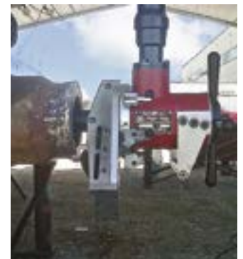
SDB end prepping pressure vessel
