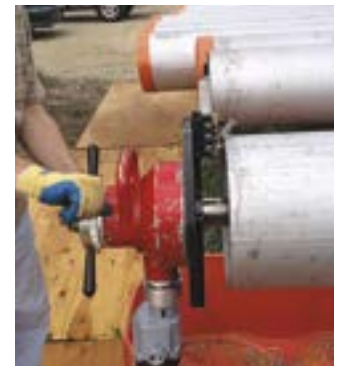
SDB pipe end preparation
