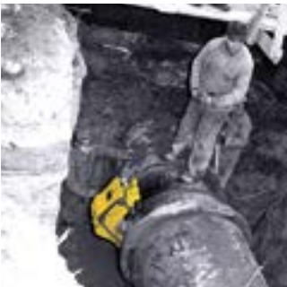
Early cutting with Trav-L-Cutter
