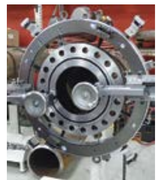
Two FFC modules simultaneously machine bolt face & record groove
