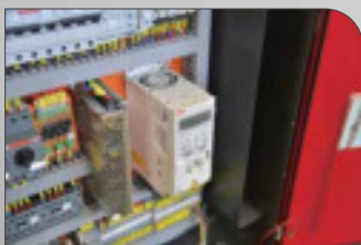
13- INVERTER (VARIABLE SPEED)
