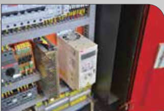
13- INVERTER (VARIABLE SPEED)
